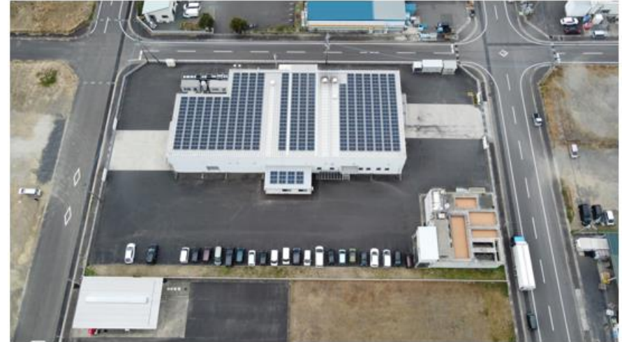
Solar power generation system at STARZEN MEAT PROCESSOR Co., Ltd., Akune Plant Processed Food Production Center
